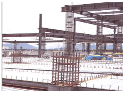
Fig. 2 Typical RCS frame
