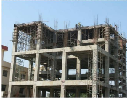
Fig. 1 Typical RC frame
